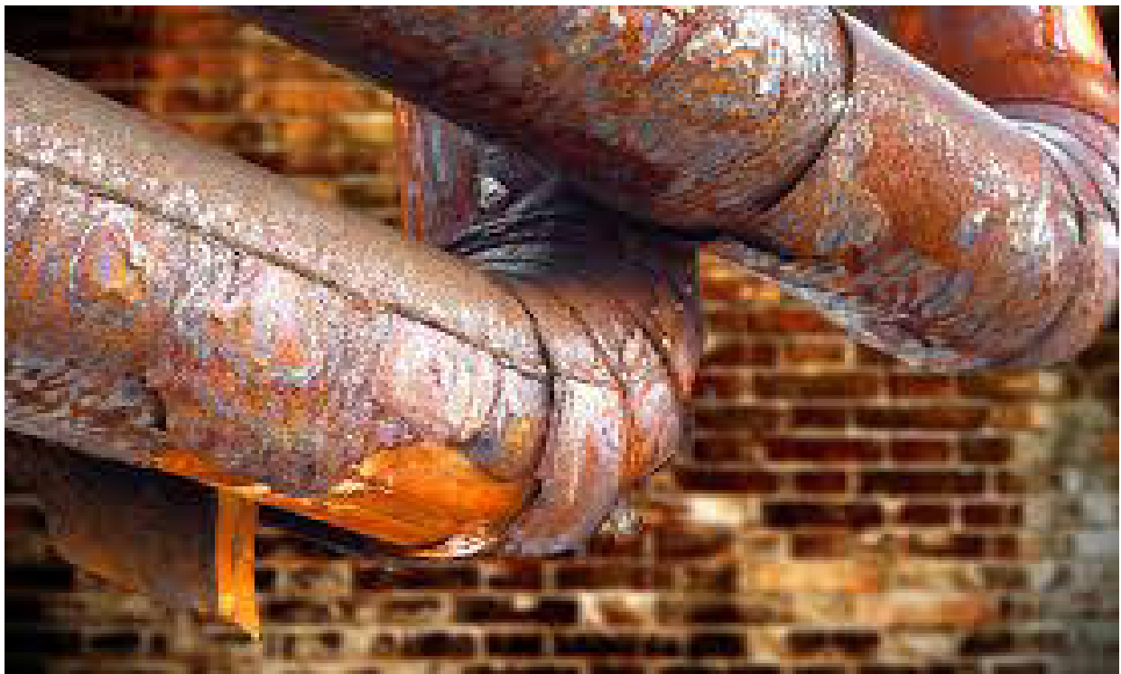
Figure.1 Different types of water pipeline corrosion during water flow.
