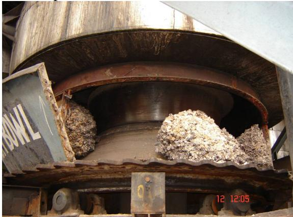
Figure 1: Ash bowl arrangement with guide roller
